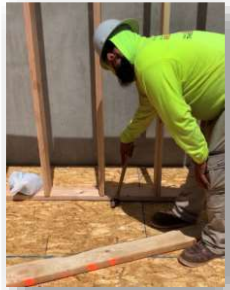
Moving Material (drywall, siding, wood)
