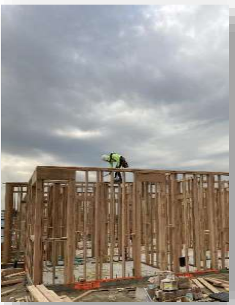
Hammering Nails (8D- 16D & Duplex Nails)
