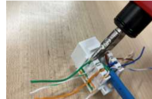
Terminate each conductor with punchdown tool.
