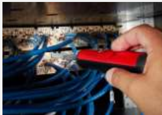
110 and 66 Blocks and Patch Panels are larger termination blocks used for connecting multiple cables , typically in data closets .
